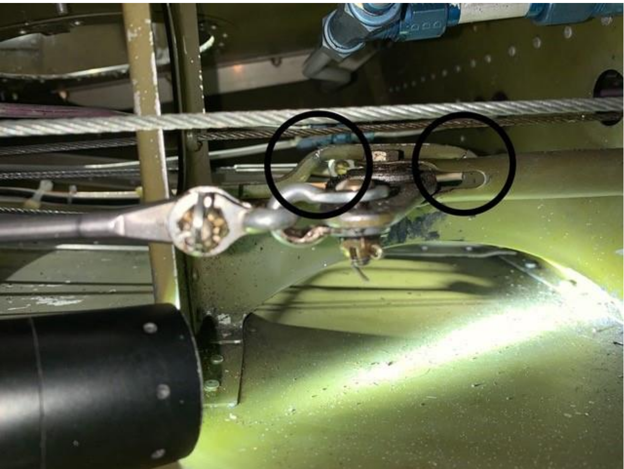
Photo 2 : Elevator Bellcrank and Bracket Assembly - Cracks found in upper bracket P/N 0411290.
