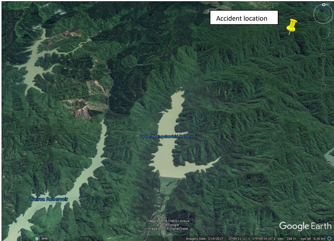
Figure 4: Aerial view of the Wairoa Reservoir, Upper Mangatawhiri Reservoir and accident location (Google Earth).
