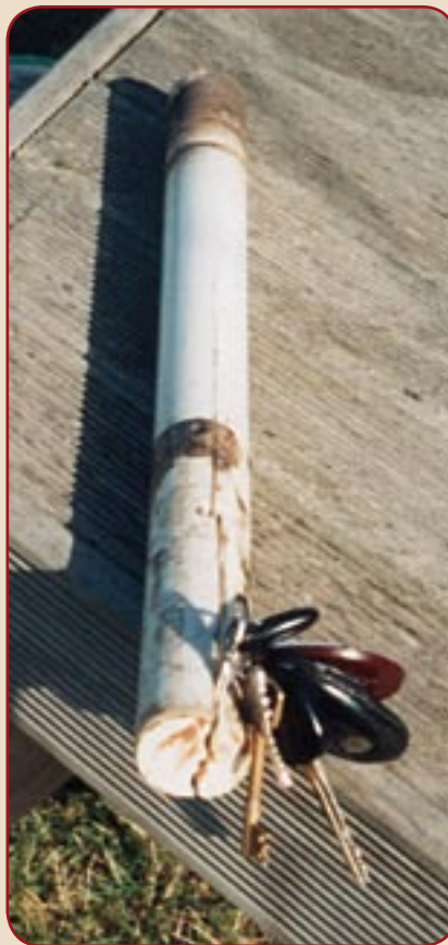
The fibreglass landing gear leg with a very noticeable longitudinal crack in it which began under the sleeve. The crack was large enough that a key could be inserted into the upper end of the crack.
