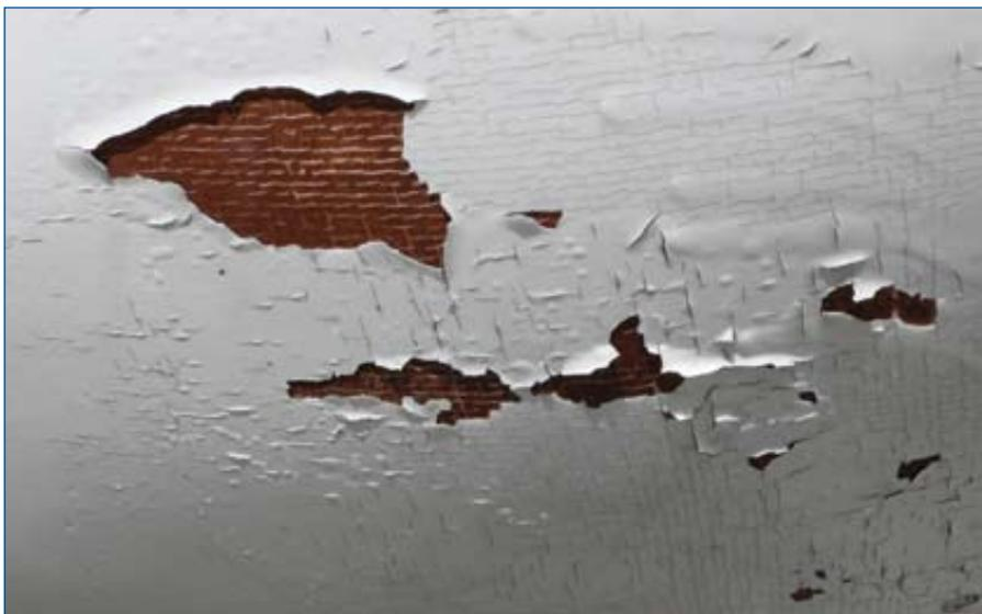
Poor preparation and painting caused this blistering.
