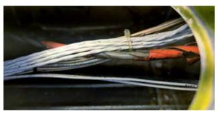
// Incorrect routing of additional wiring has a pipe running through the middle of the wiring bundle.
