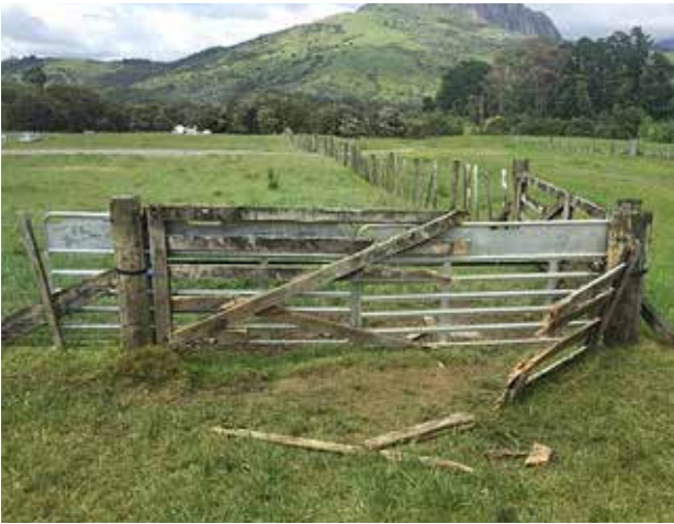
// The replacement gate, and the remnants of the original.
